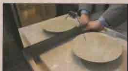
Lavatory: The lavatory has a raised, flat center surface that sits flush with the outer edge, and a higher level from which water cascades.
