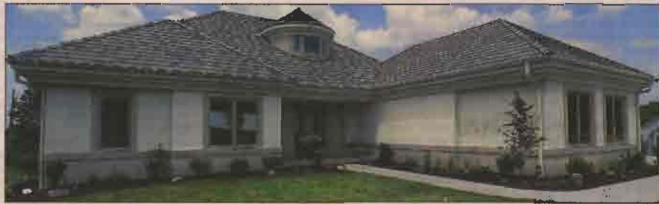
Many helped: More than 30 businesses contributed to the 3,030 square feet of living space for the Alliant Energy PowerHouse in Newton.
